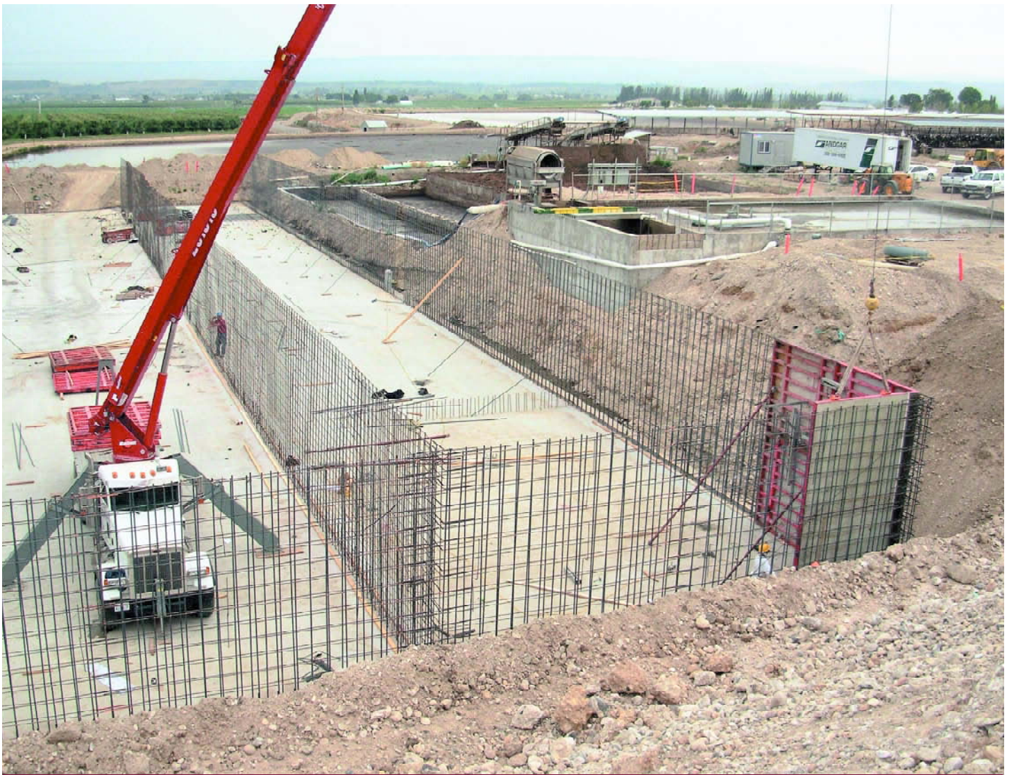
Forms are constructed to channel the flow of manure at the DeRuyter Dairy methane gas facility. Although this operation is not owned by a cooperative, this technology is well adapted for cooperatives to pursue.
